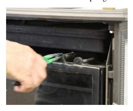
3. Use a 7/16" wrench or nut driver to remove the glass retainer at the bottom front of the firebox.
